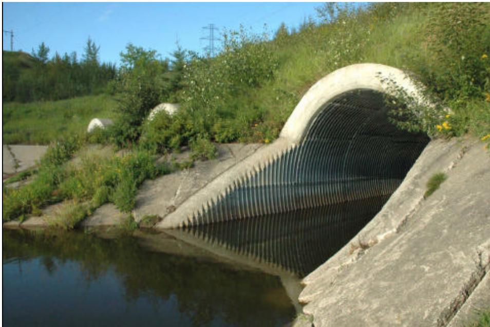
The Sturgeon River ends at this earthen embankment near Fort Saskatchewan, flowing through three large metal pipes. The embankment is roughly two stories tall.
